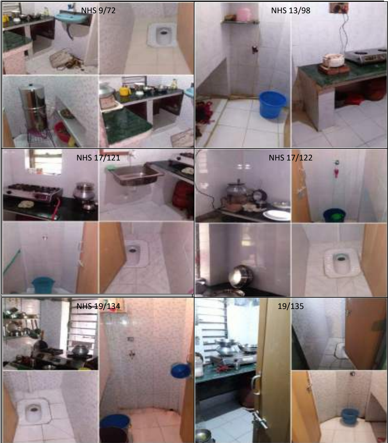
INSIDE BLOCK REPAIRING WORK OF NHS QUARTERS AT R N COLONY OF SONEPUR BAZARI AREA
