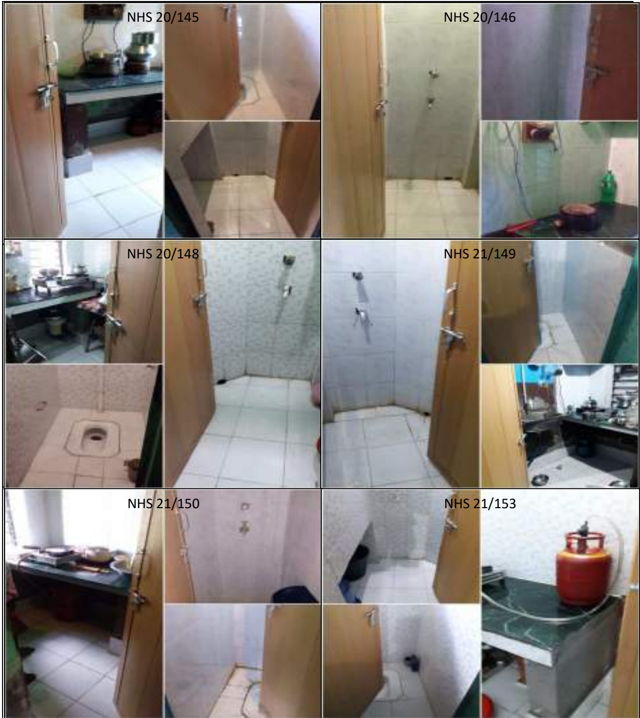
INSIDE BLOCK REPAIRING WORK OF NHS QUARTERS AT R N COLONY OF SONEPUR BAZARI AREA
