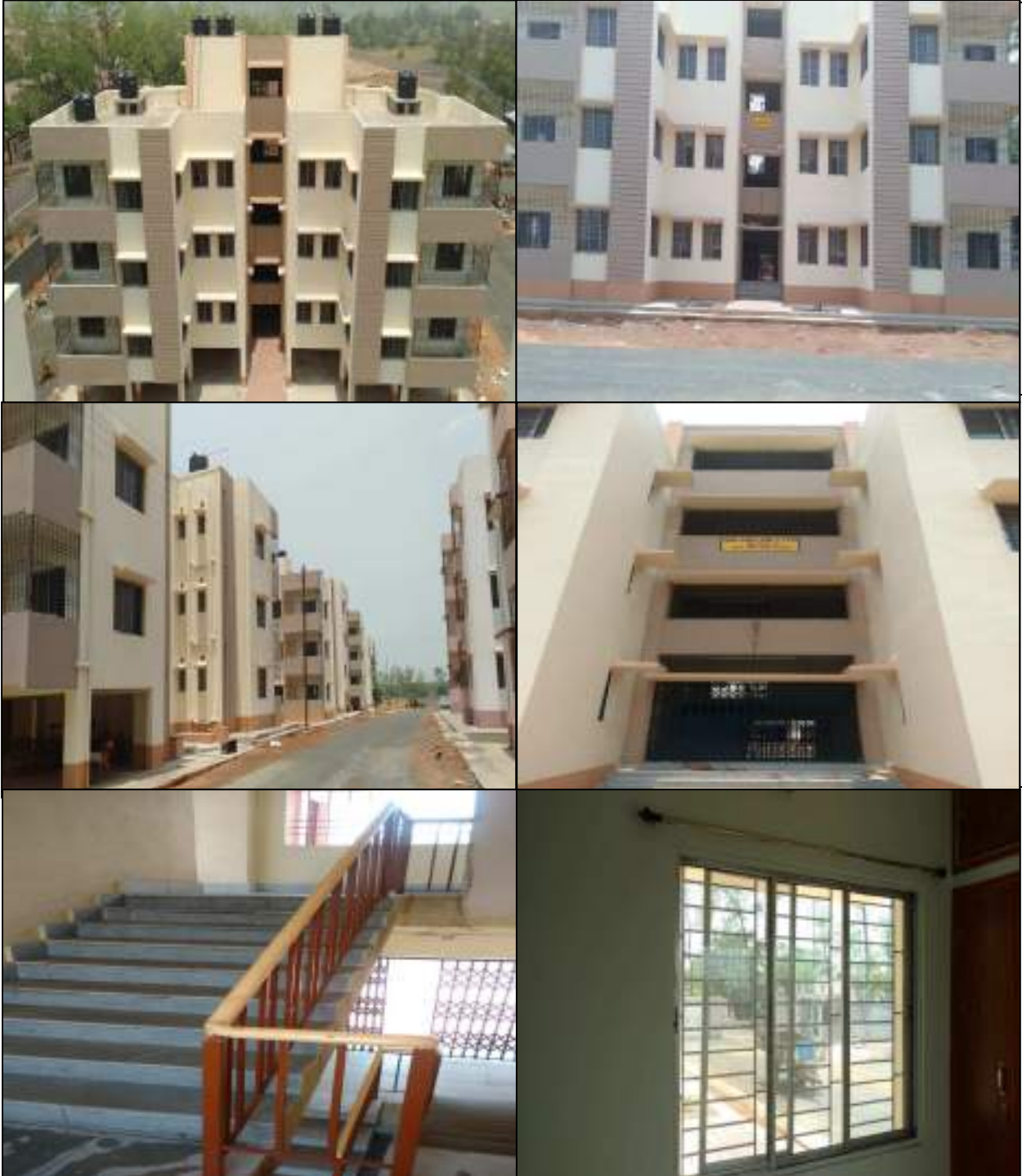
C TYPE NEWLY CONSTRUCTED BLOCK AT V N COLONY OF SONEPUR BAZARI AREA
