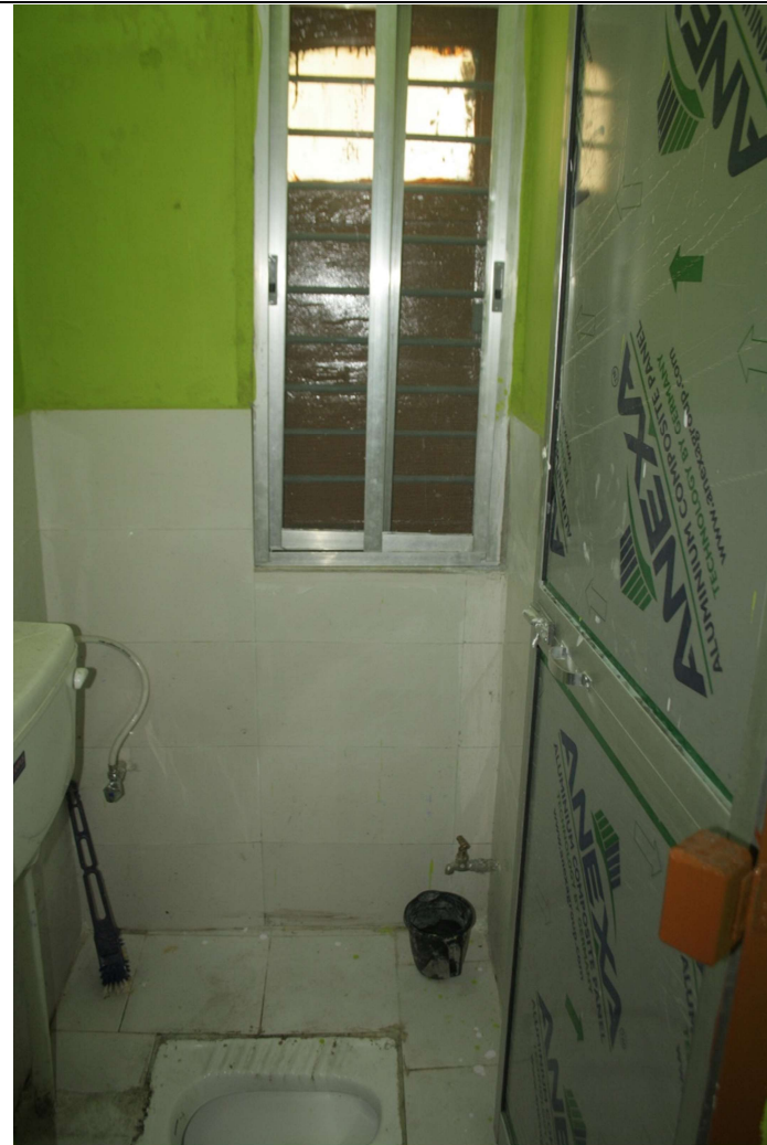
Quarter Repair at Rajmahal Area
